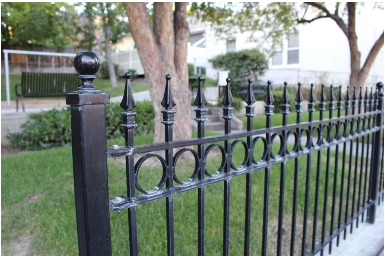
Fig. 8. Victorian-era wrought iron fence creates a formal border along the 4 th Avenue entrance frontage (Siri Vlastic, 7/30/15).
