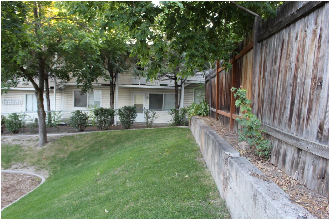
Fig. 21. View to the west standing near the northeast corner of the park. Note the chain-link and wooden fences, retaining wall and slope (Siri Vlastic, 7/30/15).
