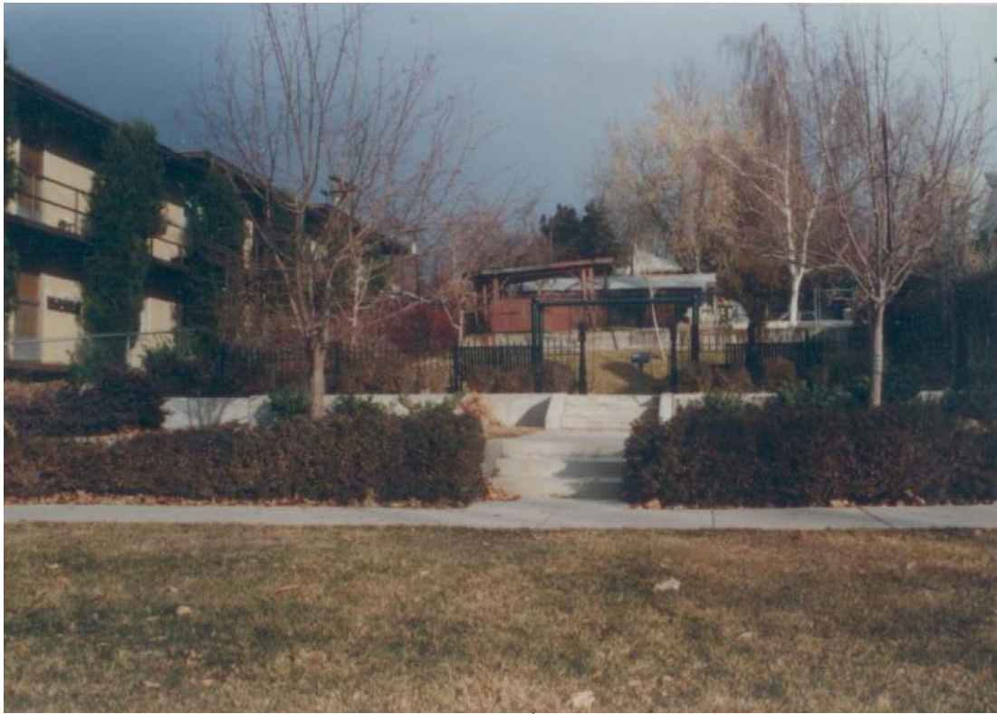
Fig. 30. Undated northwest view of the park on 4 th Avenue prior to 2009 ADA improvements. Note the iron fence located after the second stair landing instead of after the first (Salt, Parks).
