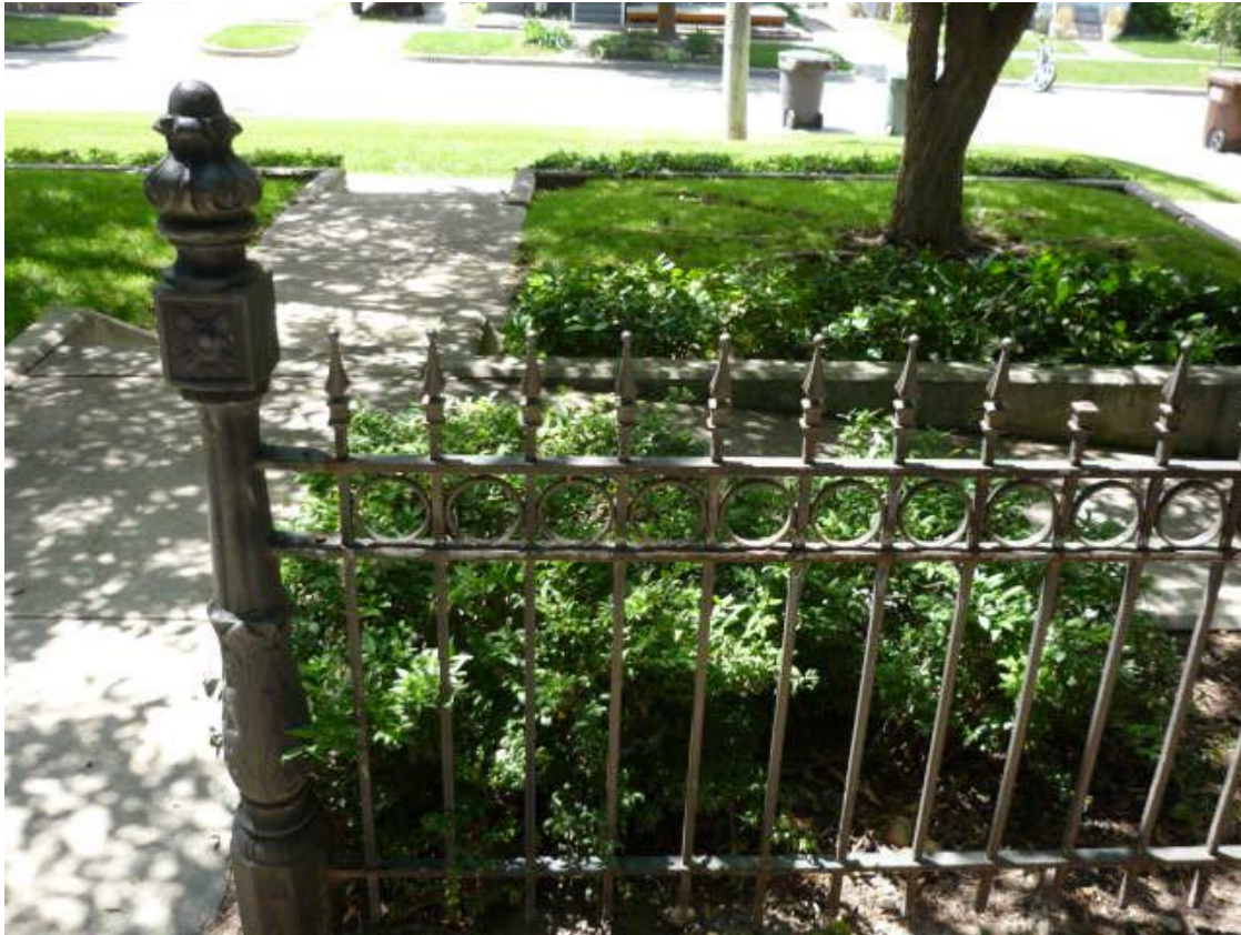
Fig. 34. Victorian-era wrought iron fence detail in 2009 before it was coated black (Landscapes 6).
